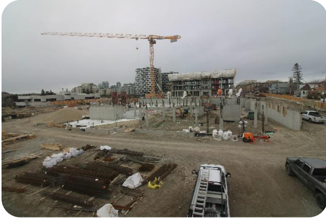
Construction continues on West Tower
