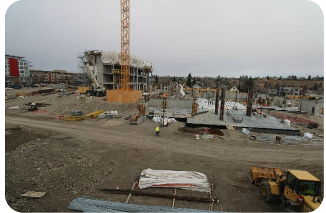
Level 4 is poured forming the 5 th floor slab
